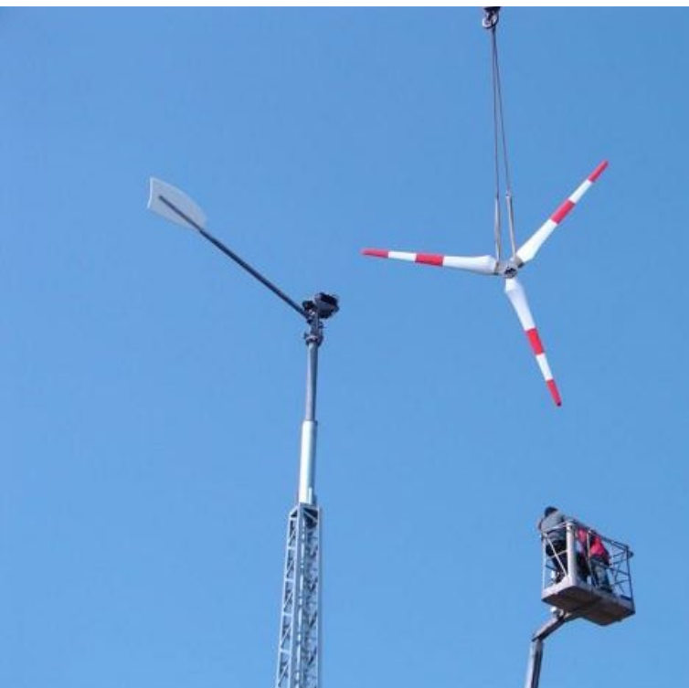
Picture 8: Separate mounting of the machine support and rotor onto a freestanding mast with crane and lifting platform. On sufficient ultimate load of the lifting platform the parts can also be transported to the top of the mast separately.
