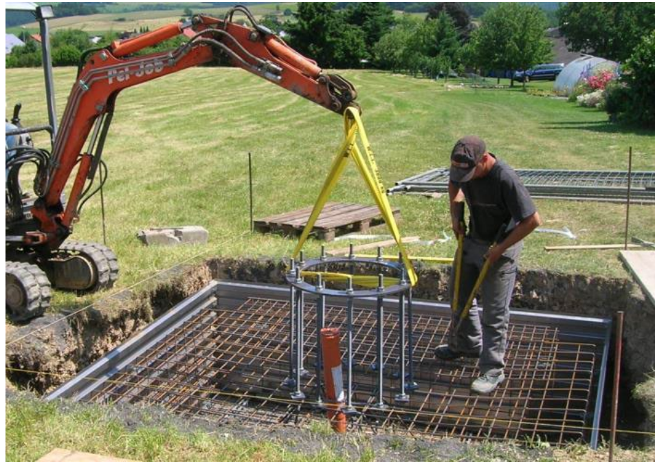
Picture 2: Installation of the lower flange (anchorage) into the fundament with the inner empty conduit for the generator connecting cable
