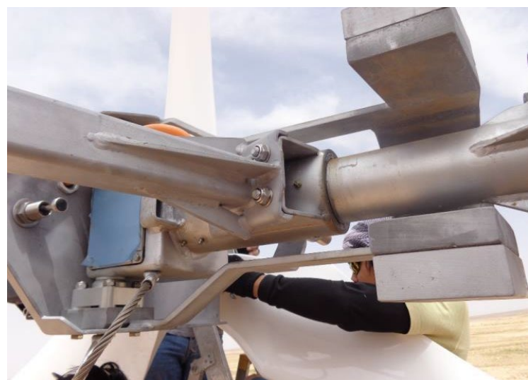
Picture 5: Pipe to the wind vane screwed to machine support. The 4 screws M12 are tightened with 50 Nm.
