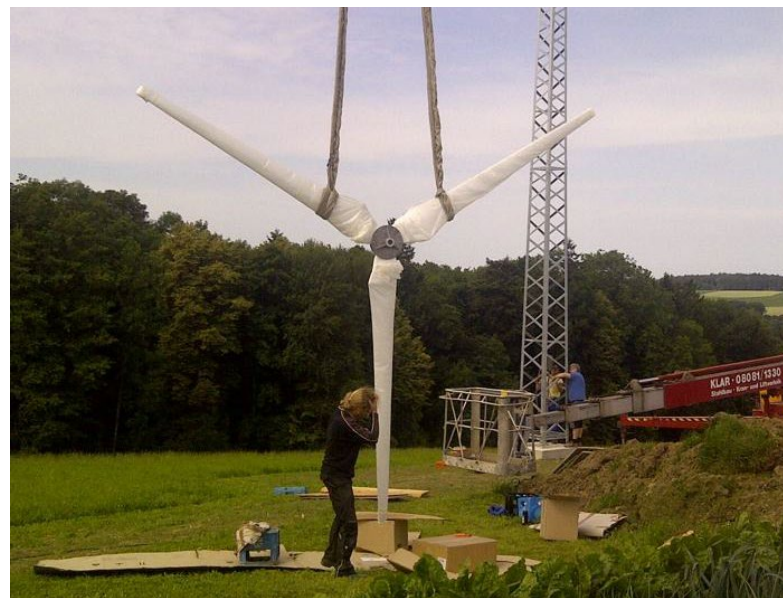
Picture 7: Pre-mounted rotor
