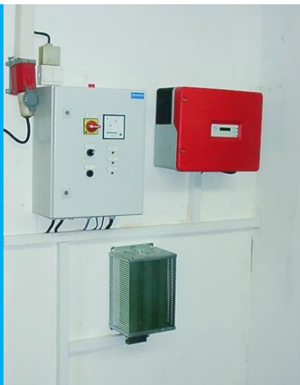
Picture 5: Upper left: control cabinet, right-side: Windy Boy from the company SMA, bottom: braking resistance
